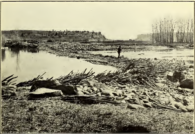
FIG. 2.—A BRUSH DAM ON THE YELLOWSTONE RIVER.
